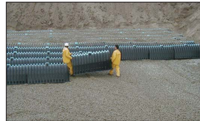
After - In a project led by TreePeople, the schoolyard was redesigned to replace much of the asphalt with landscaping, and includes an underground infiltration field to capture and recharge all of the runoff.
